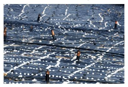
Mechanisms are laid to capture landfill natural gas (LFG), which is either piped out or flared off.
